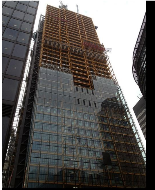
Fig. 1 Leadenhall Building under construction
