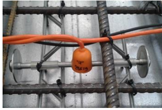
Fig 5 Example of smart-embedded building sensor
