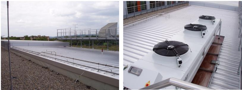
Fig. 2 Passive infrared night cooling fields (left), re-cooling unit and PINC fields (right).
