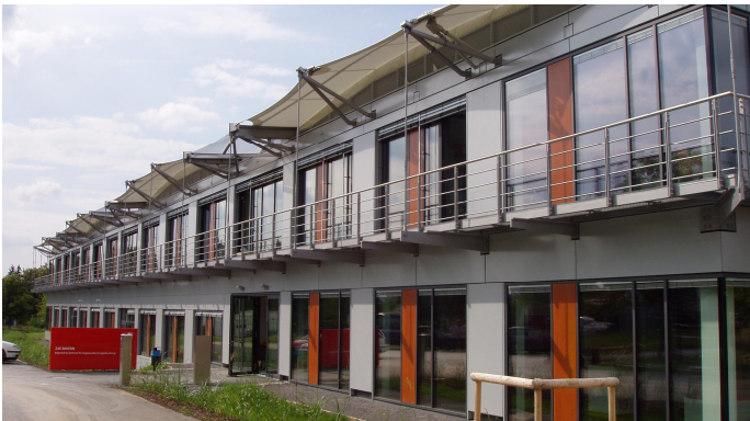
Fig. 1 The demonstrator building energy efficiency center (EEC) in Würzburg, Germany.
