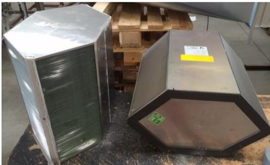
Fig. 4: Two HRV plate heat exchangers
