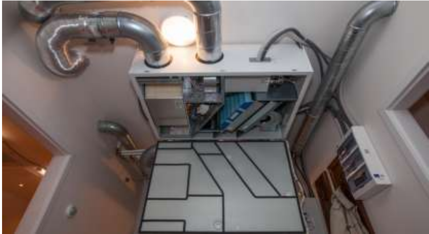
Fig. 5 Split system with recuperation and humidity control
