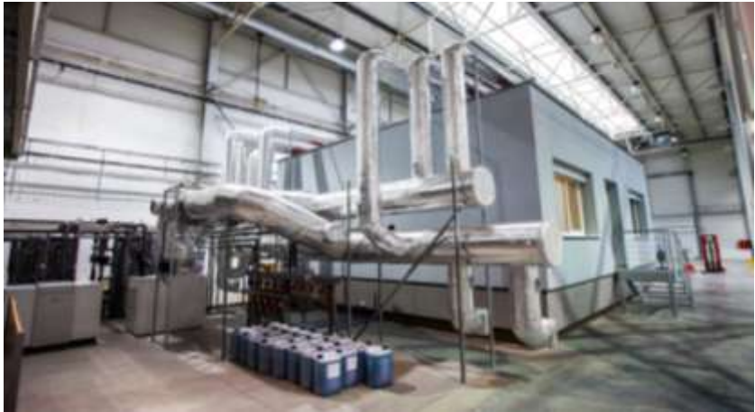
Fig. 3 The consumer model showing the heat pumps for the climate chamber (not-shown) (Photograph by Grul, R.)
