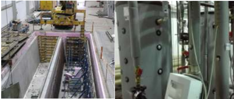
Fig. 2 Left: Insulated long-term heat storage tanks under construction with operating temperature between 15-85 ° C; Right: Short-term heat and coolth stored in 1,000 litre tanks
