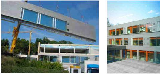
Fig. 2 Prefabricated elements for the 3<sup>rd</sup> floor in the secondary school of Schwanenstadt, with bottom metal frame, deviating the 3<sup>rd</sup> from the lower floors because of fire precaution reasons (Sources: PAUAT Architekten)
