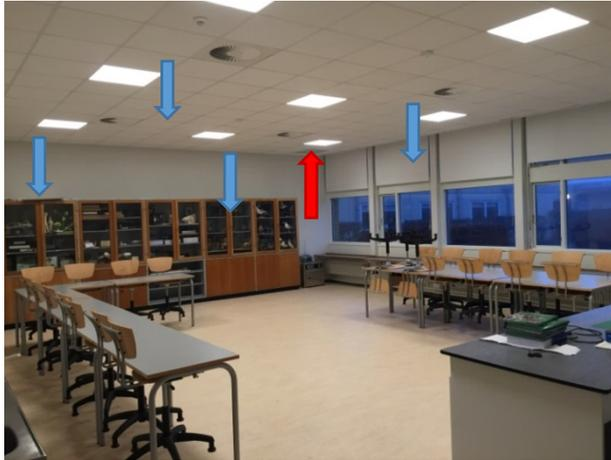
Fig. 3 Photo of classroom #2 with four swirl diffusers in the ceiling.
