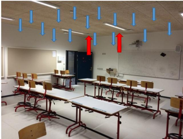
Fig. 2 Photo of classroom #1 with a diffuse ventilation ceiling. Three exhaust grilles are placed in the ceiling in a line parallel to and above the white board. Only two of exhaust are visible on the photo.
