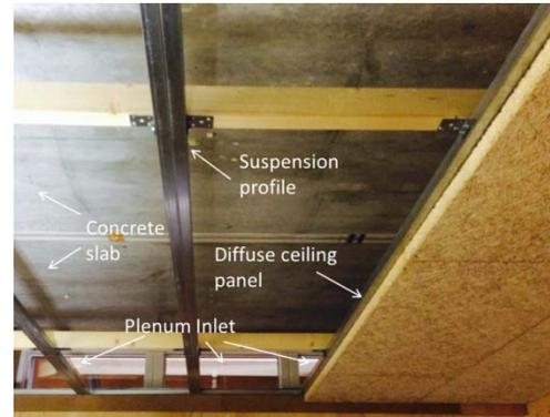
Figure 4. Diffuse ceiling panels and TABS
