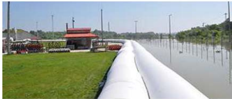
NOFLOODS SAVES GAS PLANT FROM FLOODING
