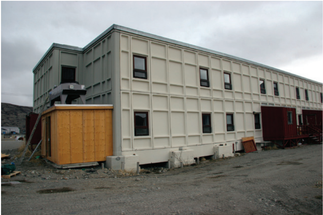
Figure 10.14 Building S385 in Kangerlussuaq suffered differential settlement of approximately 35 cm in its southeast corner after power was cut to an artificial cooling system installed below the building (photo by Thomas Ingeman-Nielsen).
