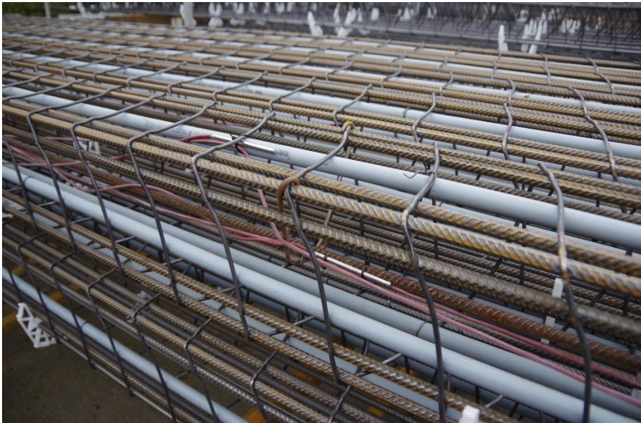
Figure 20: Pile instrumentation with Pt100 temperature sensors.
