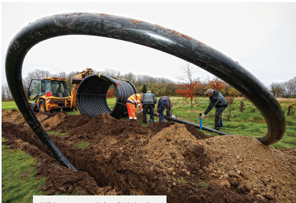
Utilizing return water in Aars district heating network, northern Jutland. Here a service line to supply a Golf Club is established.
