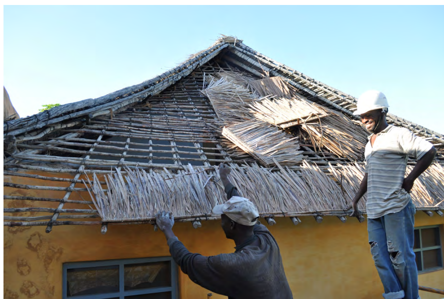
Illustration 7: Improved macuti roof construction using double tiles
