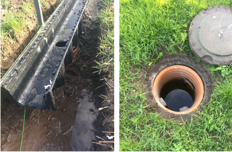
Figure 2.6. Left: Outlet from line drain to the grit chamber. Right: Grit chamber. Two inlets are seen at the bottom of the picture and one outlet towards the flow-meter at the top.
