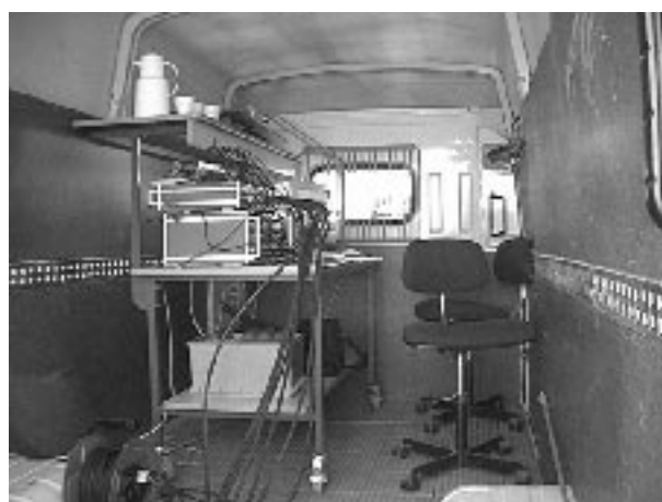
Figure 8.22: Data acquisition equipment on site.
