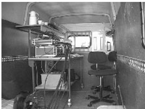
Figure 8.22: Data acquisition equipment on site.
