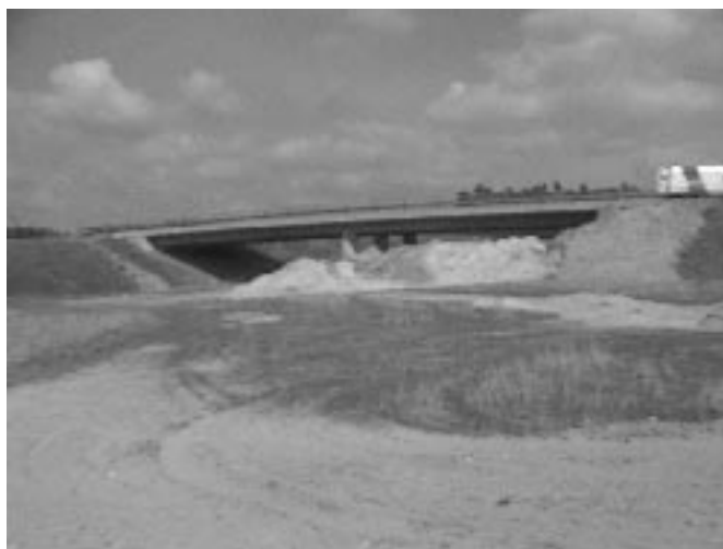
Figure 8.18: The Vestvej bridge.
