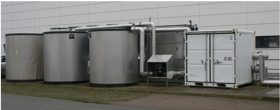
Figure 6.8: Grundfos chiller with the ice storages
