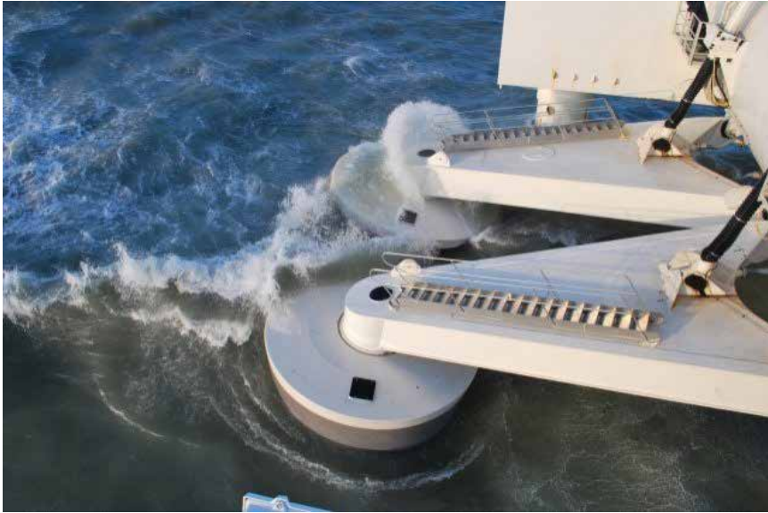
Fig. 1.1: Structural detail of Wavestar energy system, subjected to high cyclic loadings at the connection of the hydraulic cylinder and the hollow steel arm.
