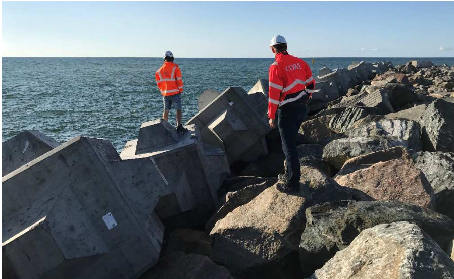
Fig. 2. Cubipod ® armour unit placed on the new breakwater in Hanstholm (summer 2018).
