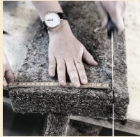
CUTTING THE SEAWEED BATTENS WITH A KNIFE
