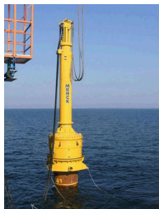
Up-close of installation of offshore piles ( www.4coffshore.com ).
