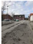
Crackled asphalt
