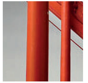
Illu.63. Galvanized steel pipe
