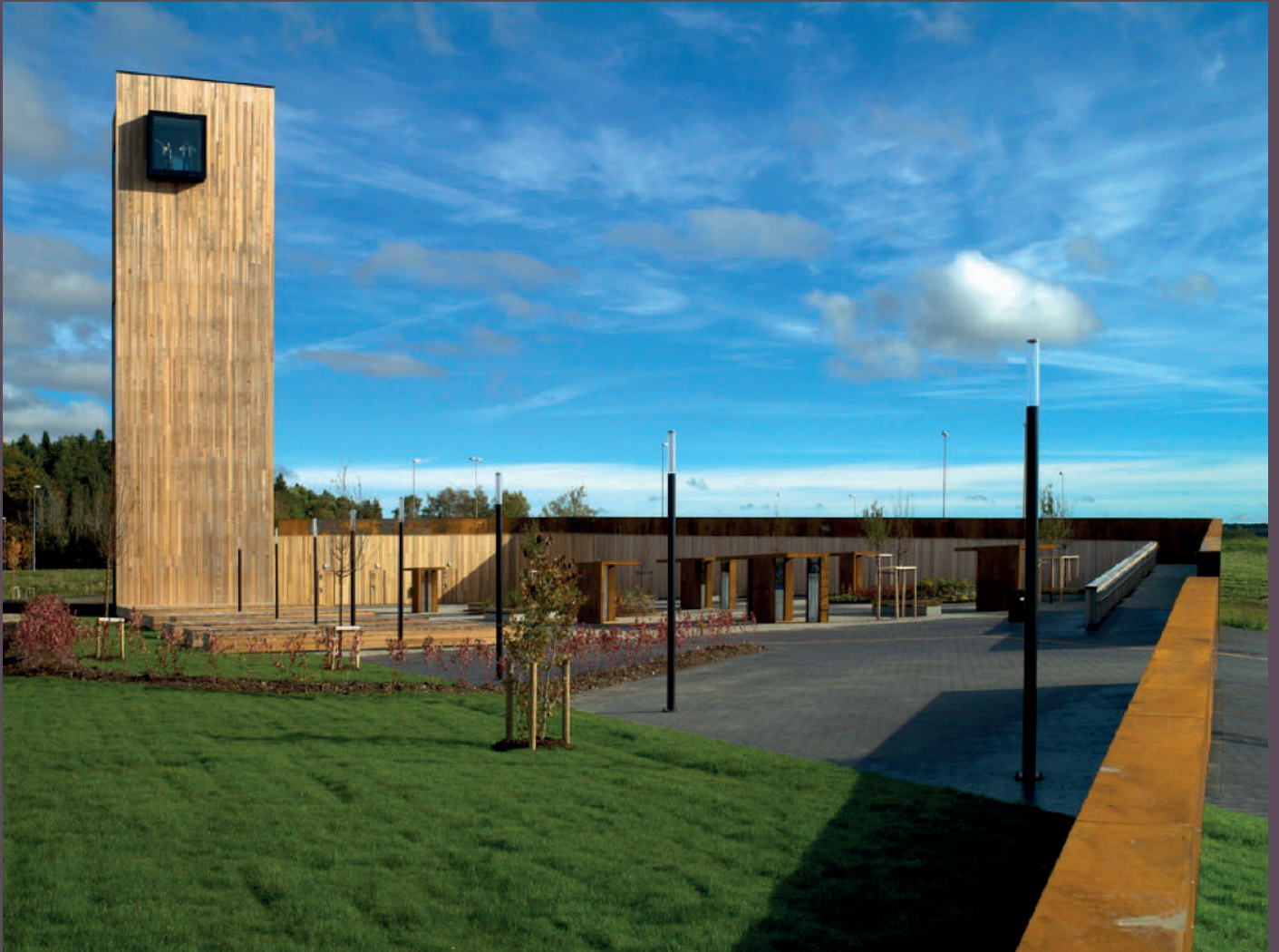
Ill. 45: Solberg Tower and rest area, Norway
