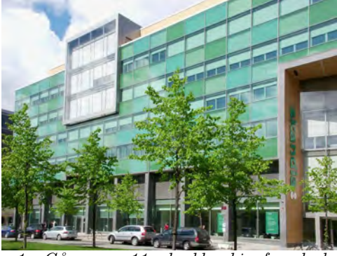
Figure 1: Gångaren 11, double skin façade building envelope
