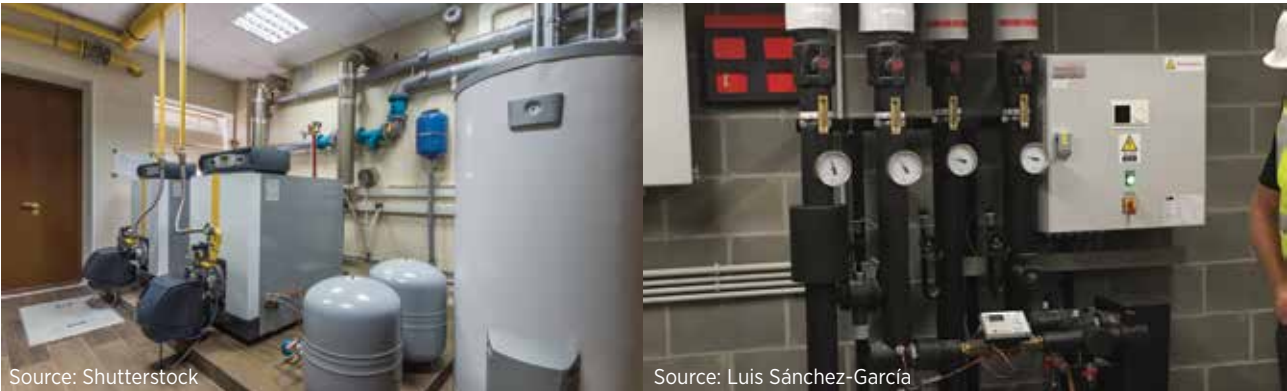
Photograph 5. Gas boilers in a gas boiler room (left) and a substation in a building in Belgium (right)
