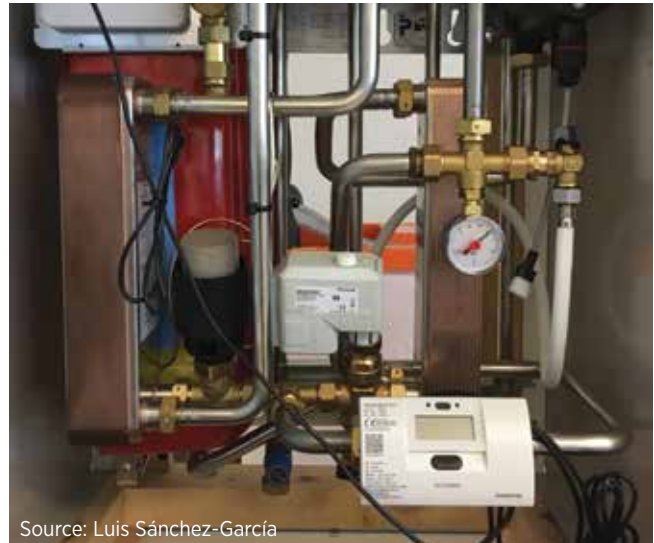
Photograph 6. Examples of water tank (left) and plate heat exchanger (right) for DHW preparation
