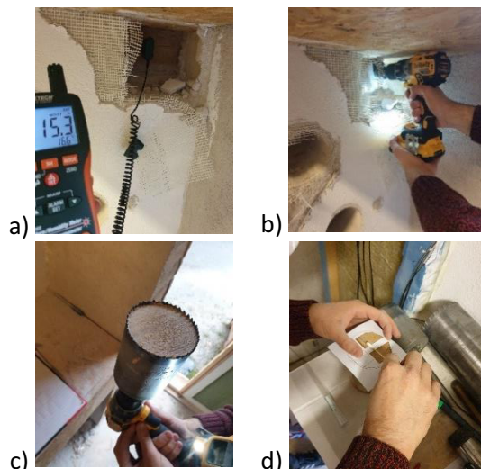
Fig. 2. Process of removing samples from the supportive wall plate. Measurements of moisture content (a) and Mycometer swabs (d) were performed on both ends of the samples.
