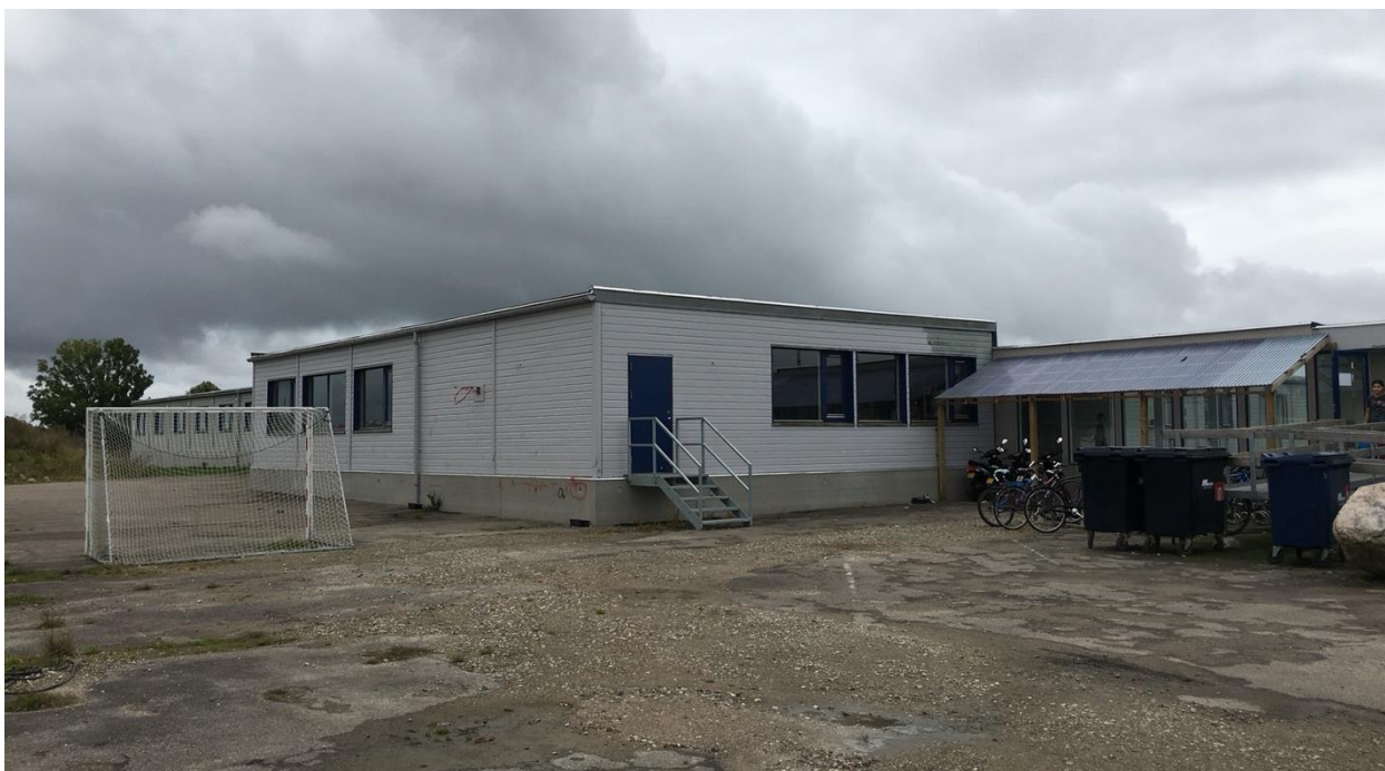
Figure 2: A temporary housing unit for refugees in Næstved in 2017. Photo: Zachary Whyte
