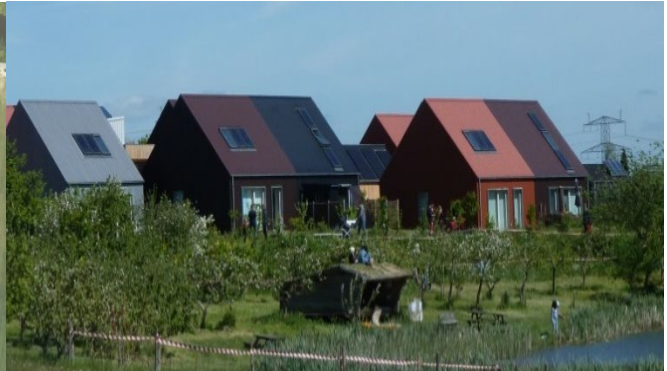
Figure 2 Houses in residential group 6
