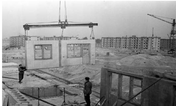
Fig.3 – Prefabricated panel construction. Source: TsDKFFA of Ukraine
