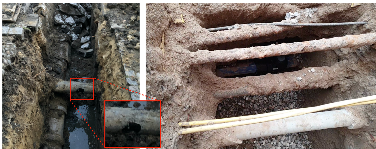
Figure 6: Damage on old utility line on the left and corrosion on utility pipes on the right.
