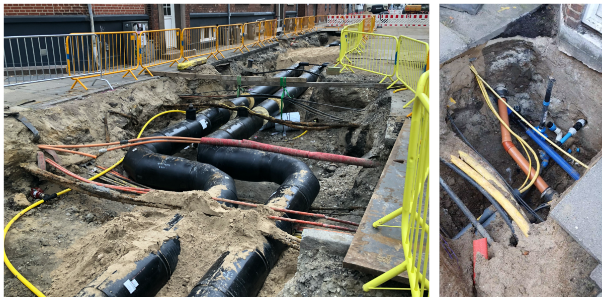
Figure 5: Big utility lines are often not explicitly described on 2D line representations on utility maps, and can sometimes be located closer to the surface than expected.
