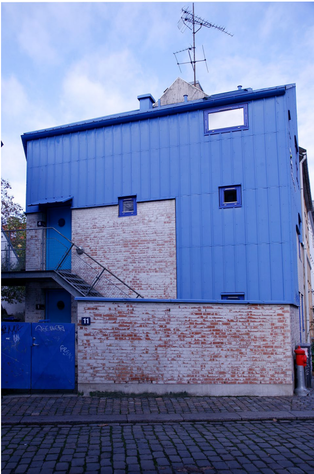
Fig. 6 Social housing The Blue Corner , 1988. Architect: Vandkunsten, Copenhagen. Photo: Louise Grønland
