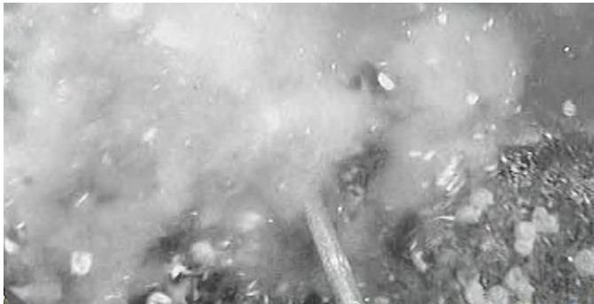
Fig. 4. Example of induced localized turbidity increase from high-pressure cleaning
