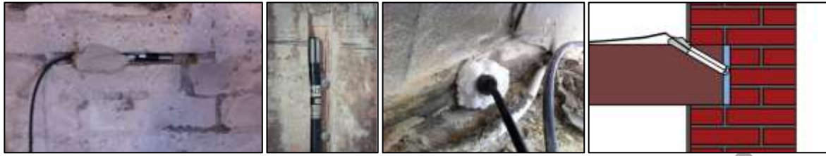
Figure 1: Sensor locations. From left to right; sensor in existing joint, purposely designed notch and in hole through beam end.
