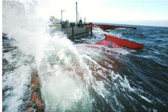
**Figure 2:** Good overtopping occurring on the Wave Dragon prototype in Nissum Bredning
