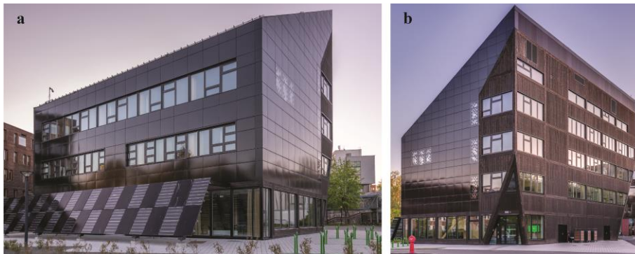
Figure 1. The ZEB Laboratory viewed from the Southeast (a), and Northeast (b). Photos:   Nicola Lolli, 2021.
