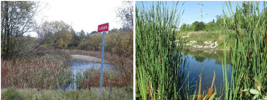
Picture 1-1 Stormwater retention ponds. The picture on the left illustrates a pond in Denmark (Jutland), while the one on the right shows a pond in Canada (Peterborough) with several inlet pipes.
