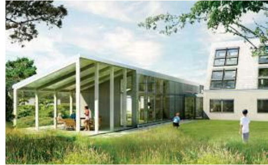
Licht Aktivhaus, 2010, Hamburg, Austria Renovated double house Picture: VELUX
