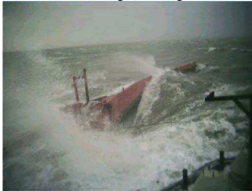
Fig. 3: View from web camera mounted to control container of large wave surging down reflector wing of Wave Dragon.
