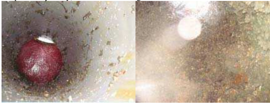
Fig. 13: The insides of two turbine draft tubes, on the left one painted with silicone paint, and on the right painting with conventional epoxy paint.
