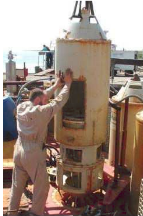
Figure 11: Reinstallation of turbine.
