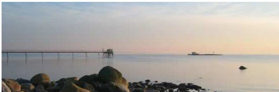
Fig. 2: The Nordic Centre for Renewable Energy's test pier, seen at sunset, with Wave Dragon floating to the right.
