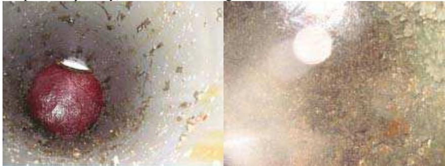
Fig. 13: The insides of two turbine draft tubes, on the left one painted with silicone paint, and on the right painting with conventional epoxy paint.
