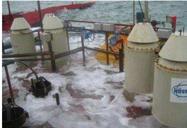
Fig. 11: Turbines in the reservoir of the prototype: The yellow structure in the background is the siphon turbine, the grey towers are five of the six cylinder gate turbines, and the small devices in unpainted steel are two of the dummy turbines.
