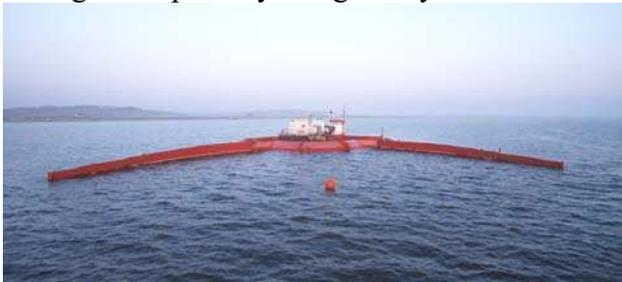
Figure 1: The Wave Dragon Nissum Bredning Prototype.
