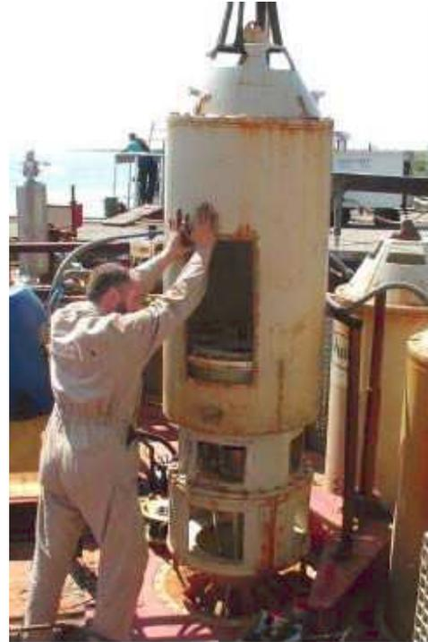
Figure 11: Reinstallation of turbine.
