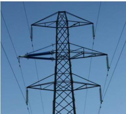
Fig. 1.3: Metallic lattice tower with composite cross-arm [17]
