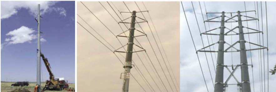
**Fig. 1.5:** 132 kV composite I-pole in Canada [20] **Fig. 1.6:** 110 kV semi-composite I-pole and full composite II-pole in China [21]
