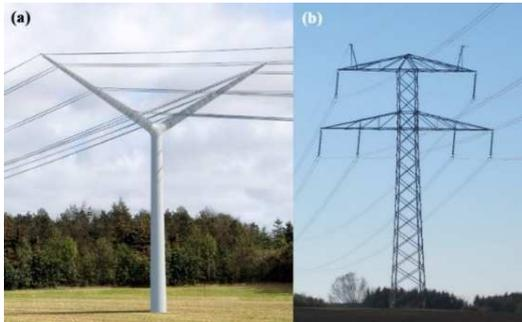
Fig. 1 Concept map of the (a) Y-shaped composite pylon and (b) Donau tower.
