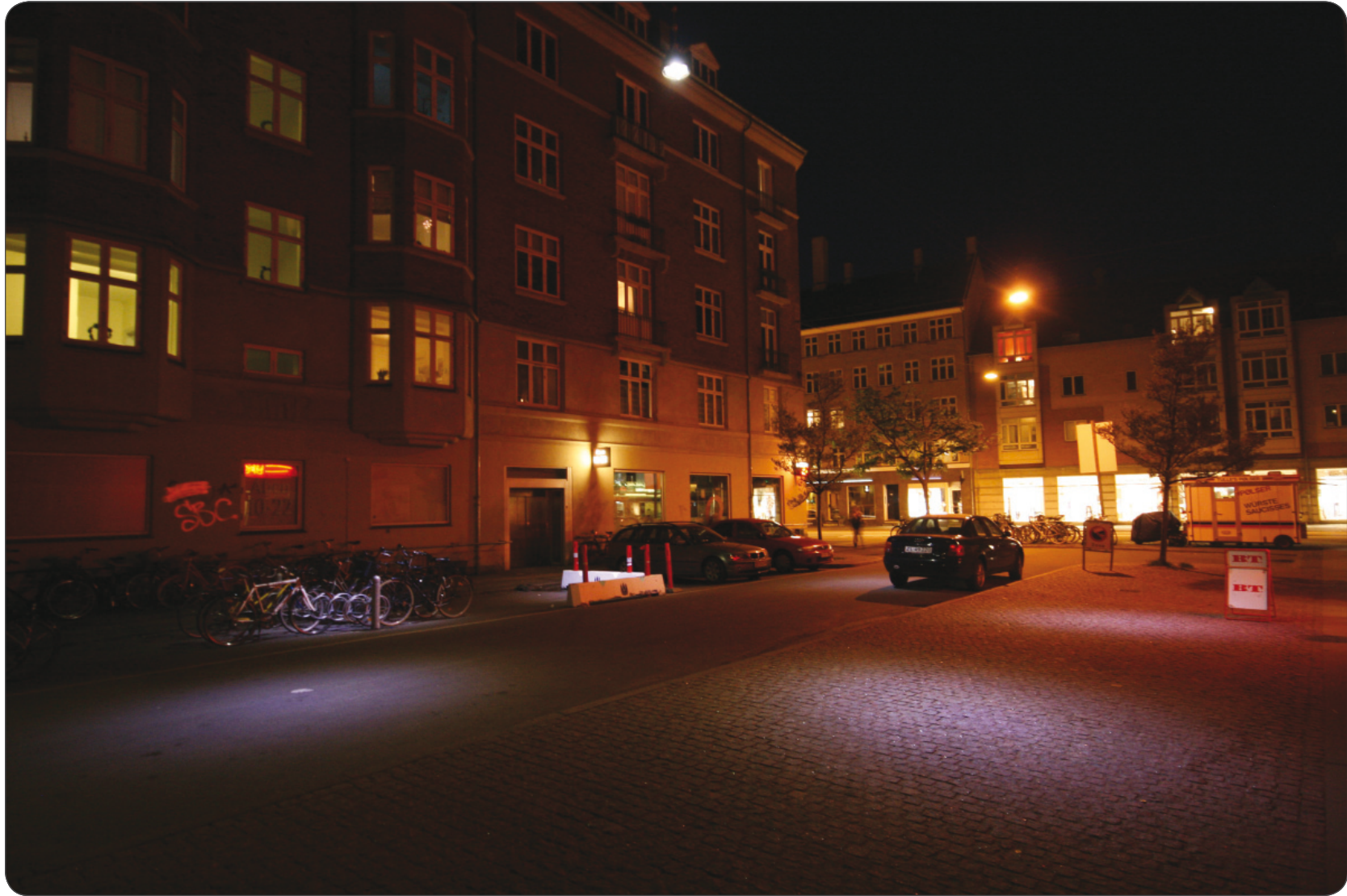
Fig. 178: New lights installed and with the old lights at the main street at the end of the road.
