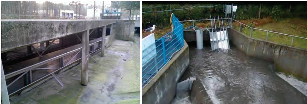
Figure 23: Photo of the internal CSO during dry and wet weather. The photos are taken from the northerly side of overflow structure towards west and east, respectively. The overflow structure are symmetric along the centreline of the inflow channel.
