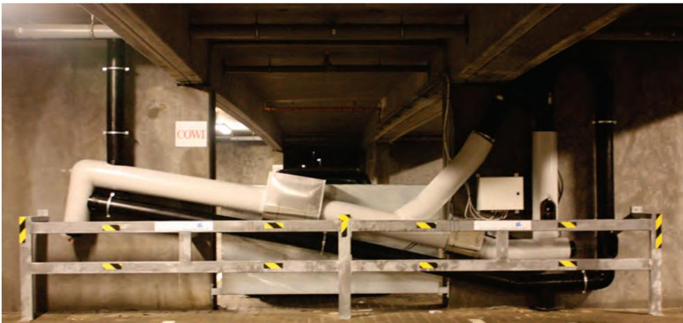
Figure 16: The runoff measurement system with heating cables, insulation and collision protection.
