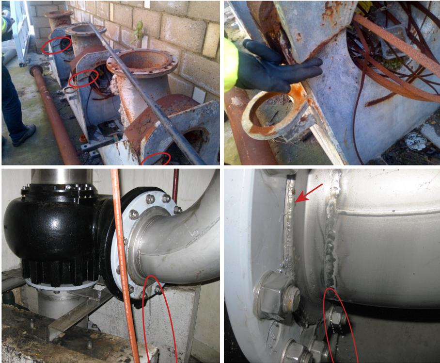
**Fig. 2.1:** Breakdown in a waste water system as a consequence of excessive vibrations. Top: Auto-coupling, on which the pump is mounted, wrecked by fatigue. Bottom: Fatigued welding in flange connection leaking water.
