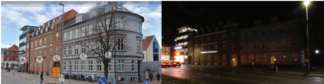
View towards east facades
