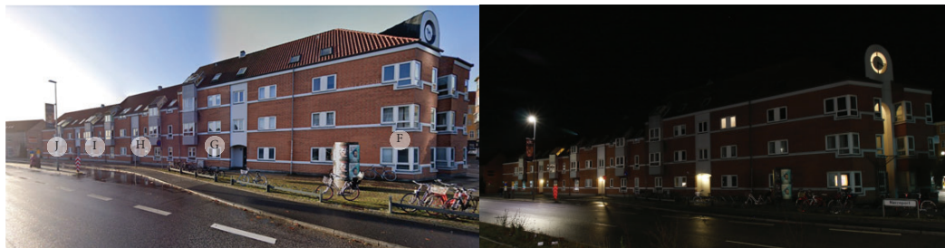
View towards west facades
