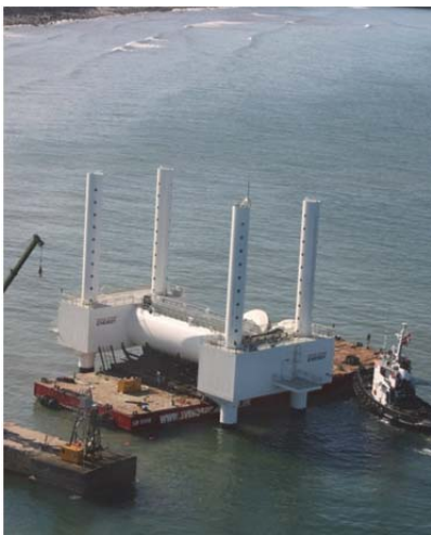
Fig. 1 Wavestar prototype. Top: Location of site (Google Earth). Bottom left: Photo of installation by barge. Bottom centre: Photo of storm protection. Bottom Right: Photo of normal operation
