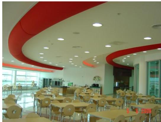
Figure 4. Vertical ventilation from openings in the ceiling.  $a_o/A \sim$  medium. The photo shows this type of flow from ceiling mounted textile terminals (KE Fibertec A/S).
