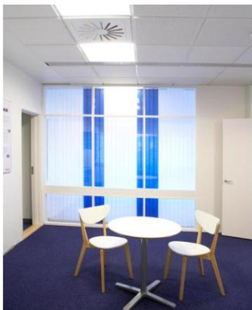
Mixing ventilation with a high location of the diffuser (Lindab A/S).
