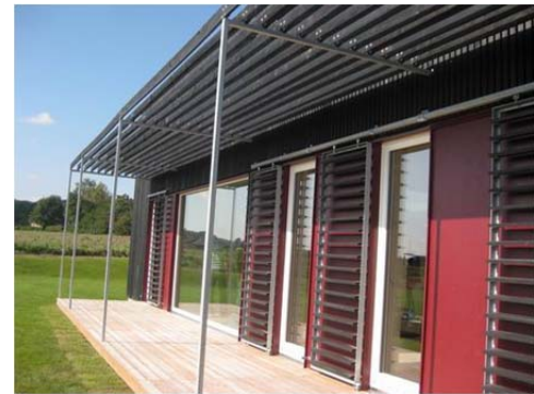
Figure 3.11: Solar shading in house 39.
