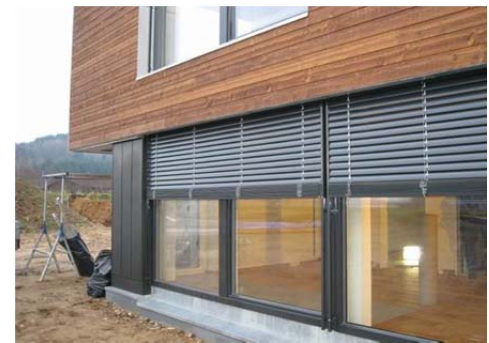
Figure 3.13: Solar shading in house 43.
