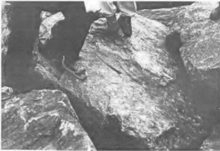
Photo from Norwegian berm breakwater
