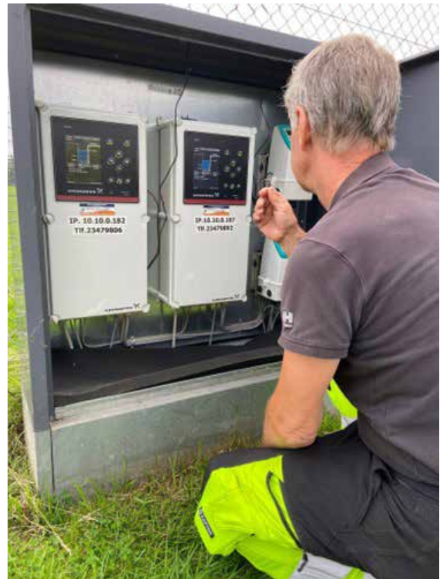
Figure 4. Brad, interacting with one of the physical controlling units supervised by the SCADA system (Photo: Jonas Falzarano Jessen)
